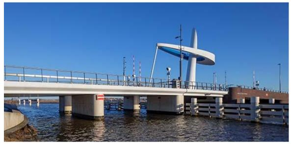
Iconic bridge for fishing village. Steel pylon and counterbalance resemble netting needle used by fishermen to repair nets. Fixed parts in concrete.
