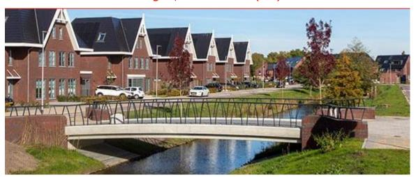
Family of four bridges designed for new housing development. Characteristic brickwork and custom-design transparent steel railing.
