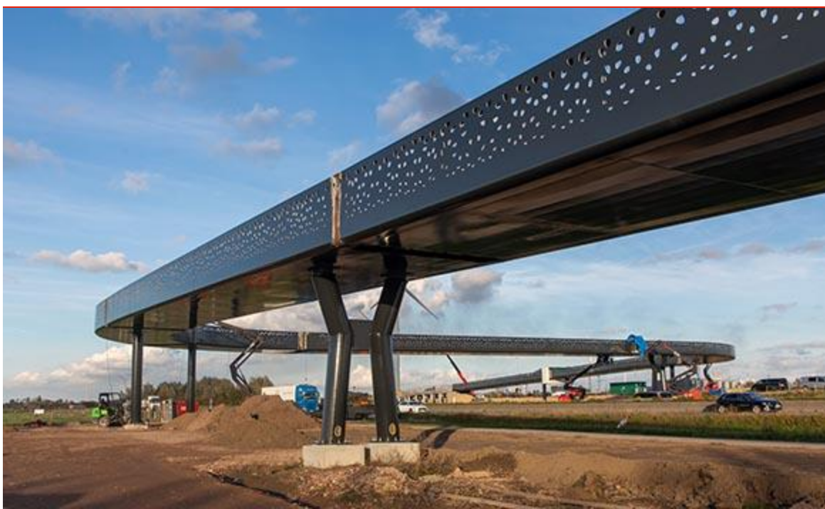
Three large bicycle bridges across the R4 ring road north of Ghent. Slender steel structures with load-bearing U-shaped cross-section.
