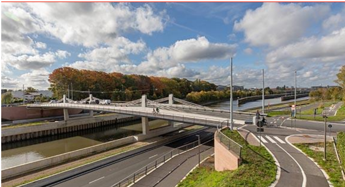
Externally prestressed concrete road bridge with cantilevered light fibre reinforced composite bicycle deck. With SBE and Franki Construct.
