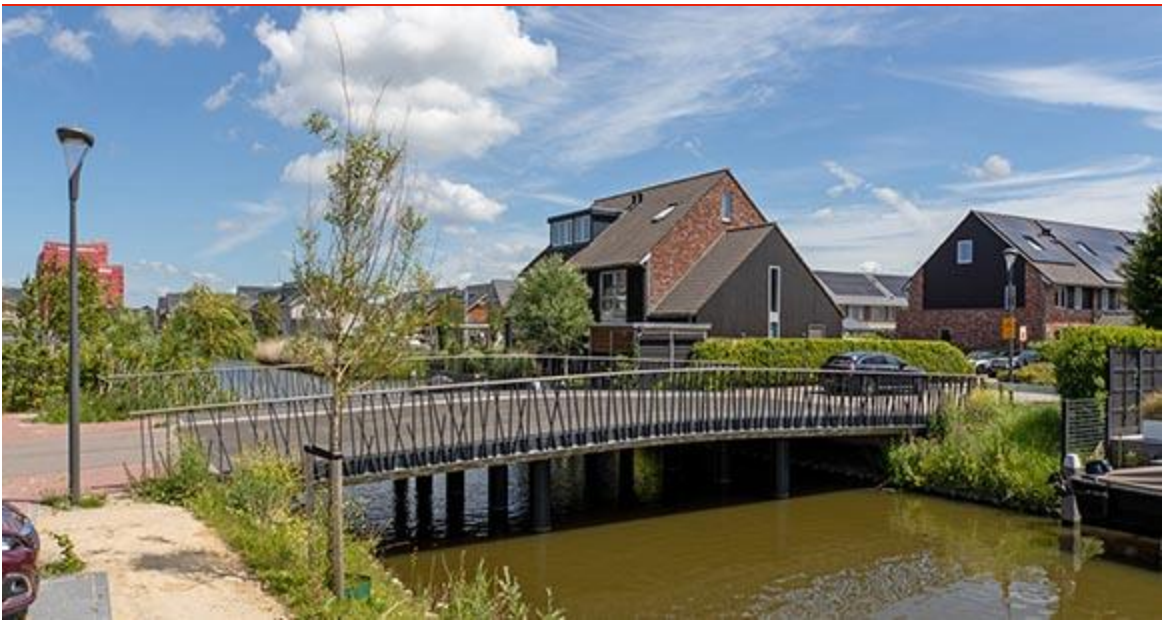
Family of bridges for new housing development. Characteristic railing design inspired by waving reed. Basic bridge structure.
