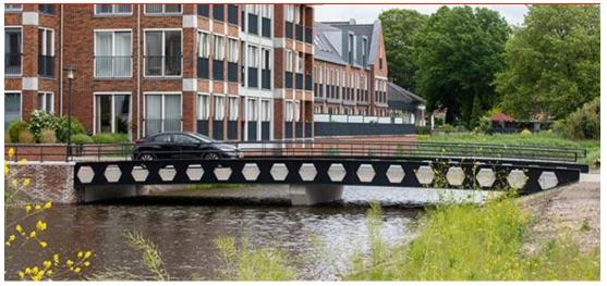
Engineering and design optimisation for basic sustainable bridge. Second hand castellated steel beams and used steel pile foundations.
